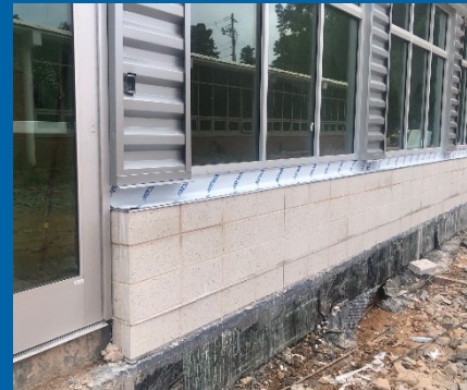
Flashing & Chamfered Block Installation
