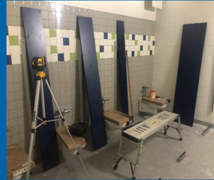
Gymnasium Plumbing Fixture and Toilet Partition Installation
